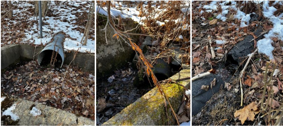
Figure 17 Culverts and drains on MU1
